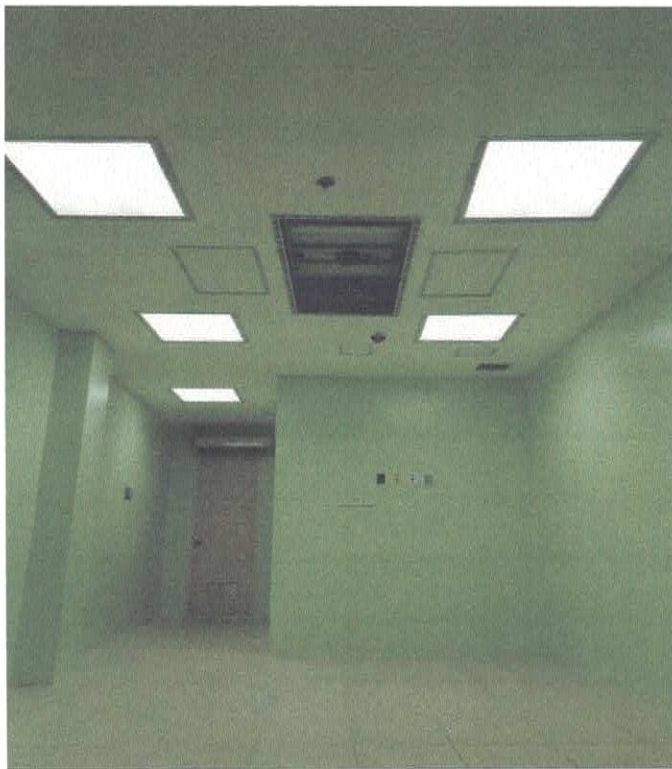
SEPTIC DELIVERY ROOM
