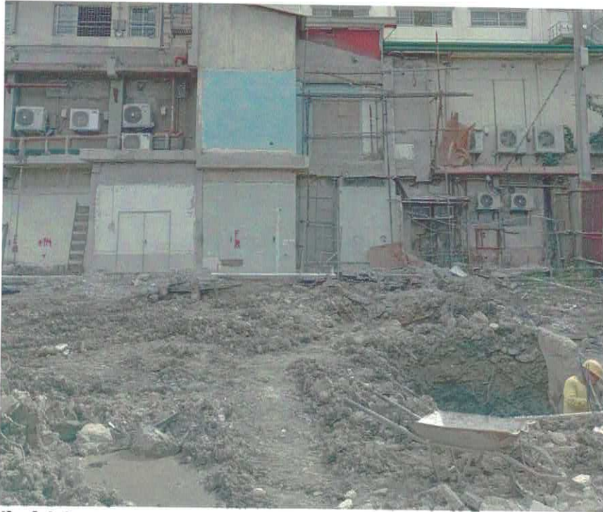
On-going pile driving
